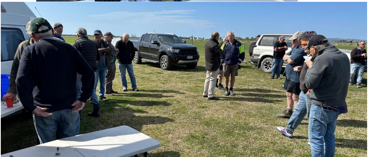
Working Bee activity followed by a late morning barbecued sausage get together to say “Thanks” to members for all the hard work demolishing the old fence line and preparing the ground for the new.
