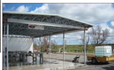
(top) Morning tea time (above) finished water blasting,
