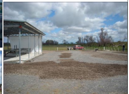
The finished carpark.
