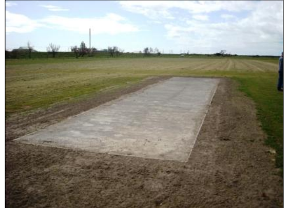
The flight-line concrete pad is now all but complete.
