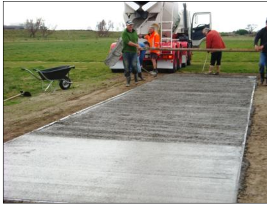
The concrete goes in.....
