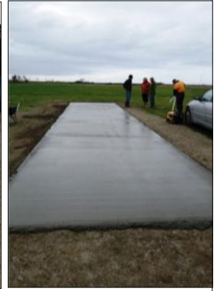
The finished result.
