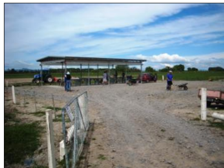
The carpark is looking better now.
