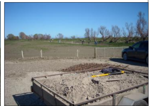
And some fencing got done too!
